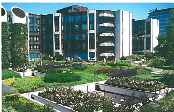
Figur 1: Intensiv takhage i United Bank of Switzerland i Basel, Sveits
